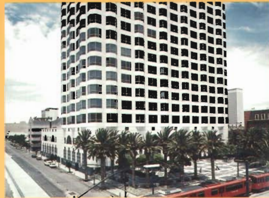
550 Corporate Center in San Diego, California
